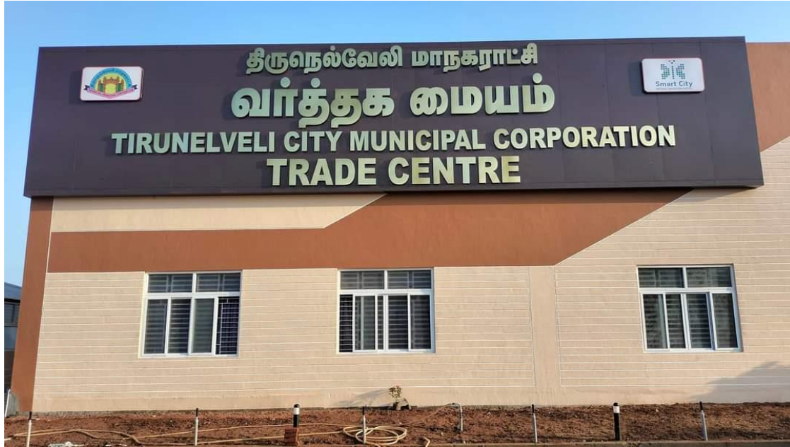
Figure 4.5 NEWLY CONSTRUCTED TRADE CENTRE UNDER SMART CITY MISSION
