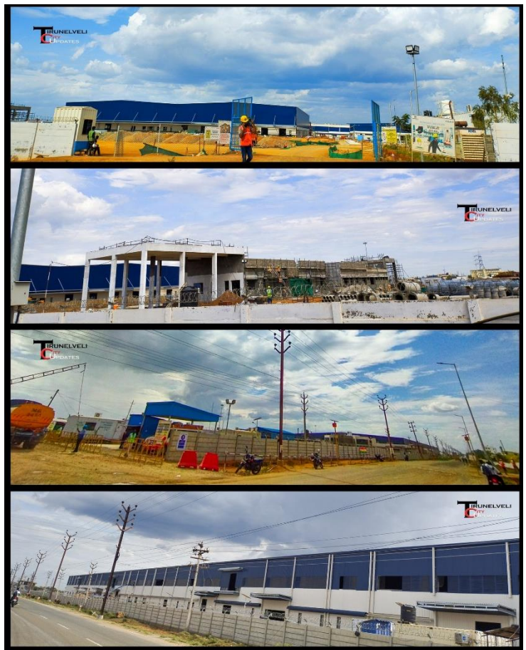
Figure 4.18 TP SOLAR UNDER CONSTRUCTION - OCT 2023
