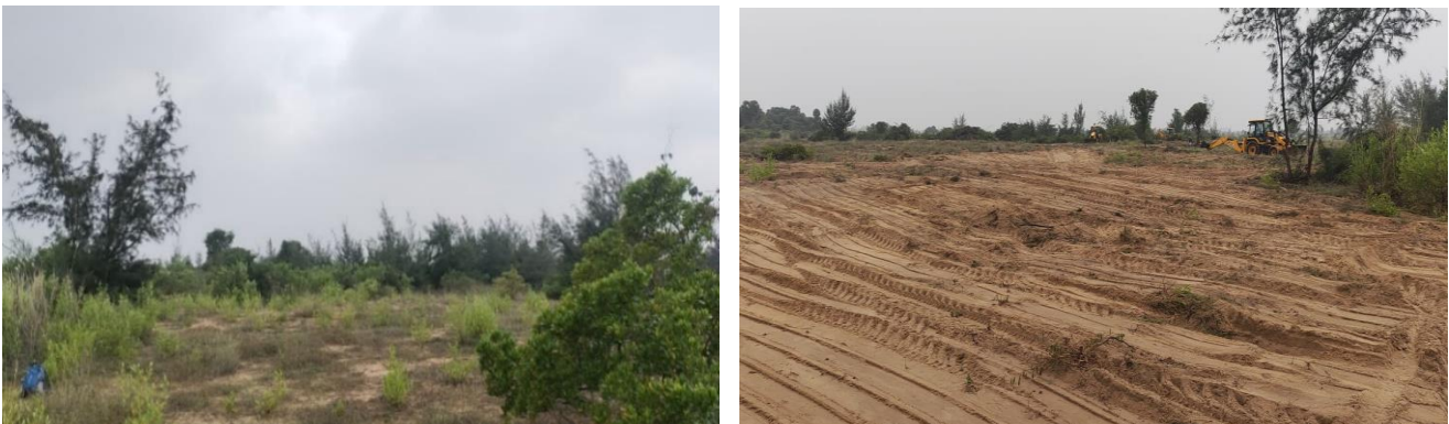
Figure 14-7 Image of the site prior [Left] and after clearance of weeds & Shrubs [Right]
