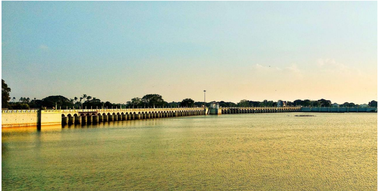
Figure 2-2 (100AD) Kallanai Dam built by King Karikalan.
