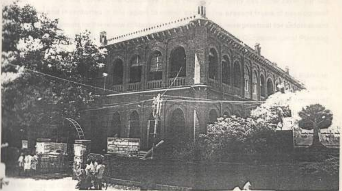
Collectorate Building, Manjakkuppam
