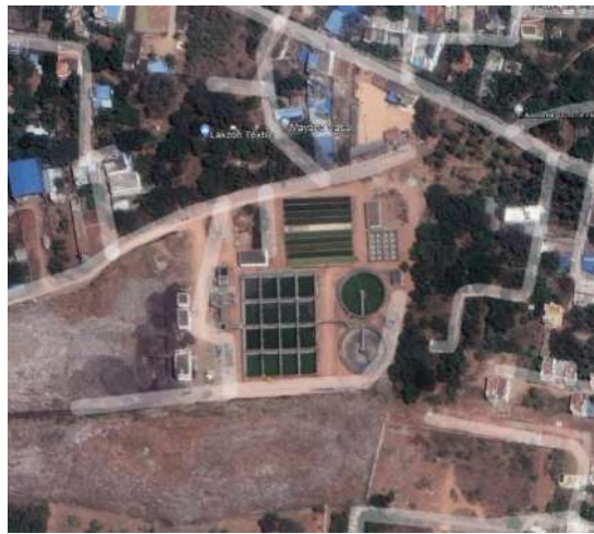
Figure 8.3 Existing STP in Nagercoil municipal corporation
