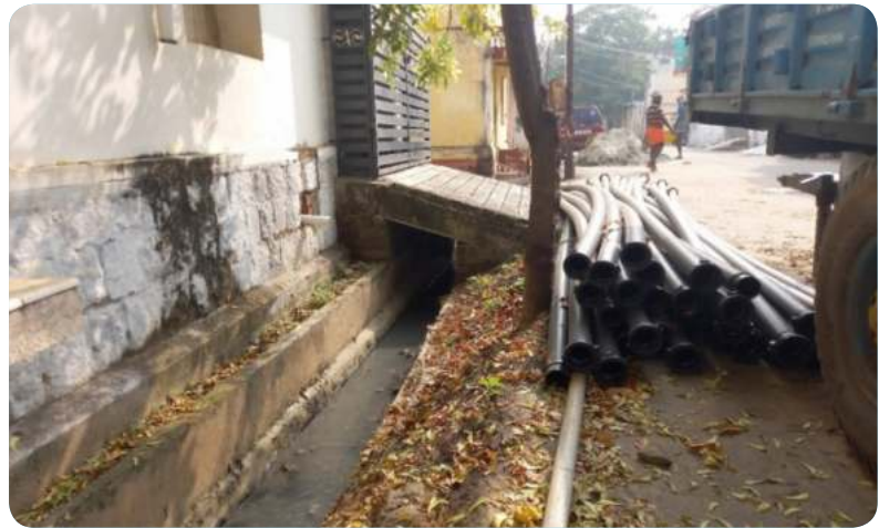
Fig 8.4: Sullage in Open Drains in Municipal Area (Near Palayapalayam)
