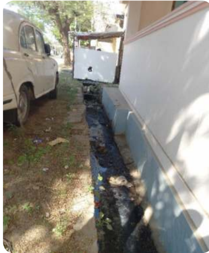
Fig 8.17: Storm Water Drain in Municipal Area (Near Palayapalayam)
