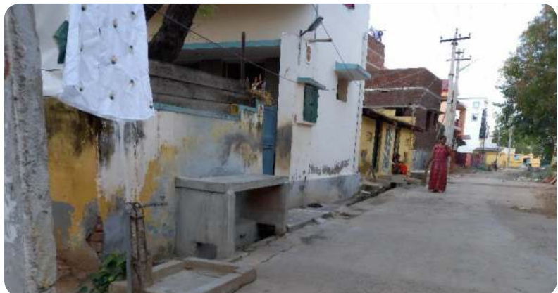
Fig 8.18: Storm Water Drain in Non-Municipal Area
