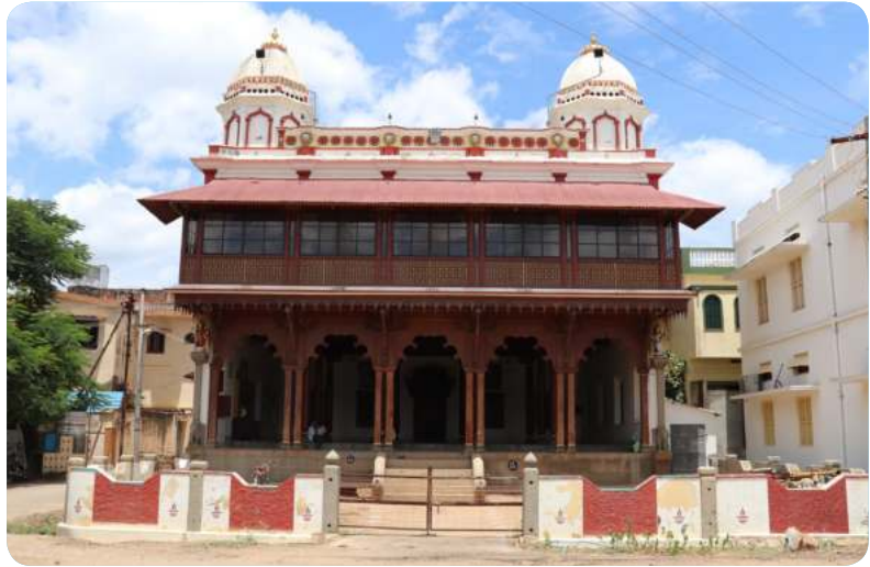
COMMON COURTYARD VIEW OF A RESIDENTIAL SUB-CLUSTER
