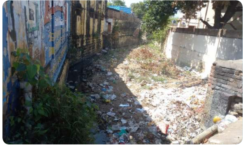
Fig 8.9: Solid Waste Dumped in Nallah in Municipal area
