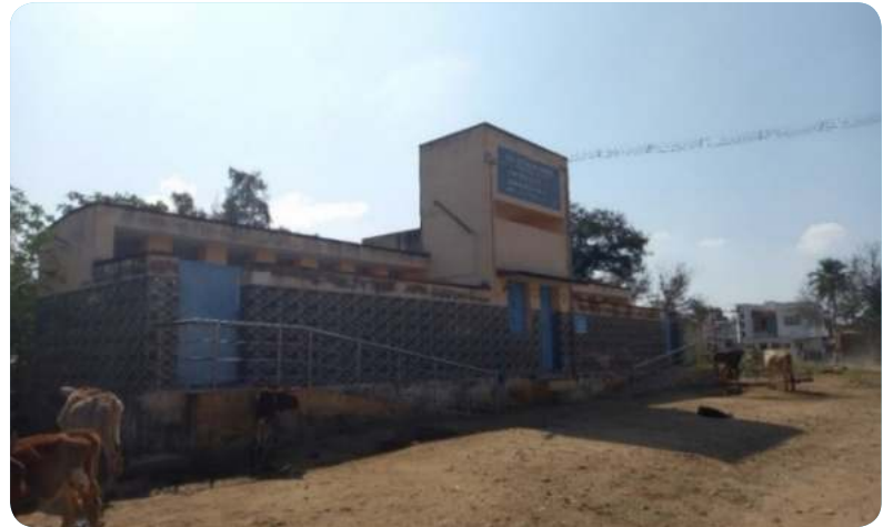
Fig 8.5: Community Toilet Block in Madasamy Kovil 60 ft. Road
